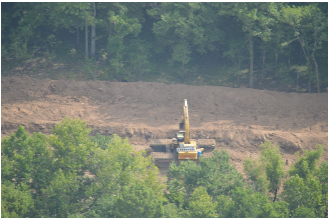
Figure 4. This photo was taken by Dean Wilson during a monitoring flight on July 23, 2018. This photo depicts the pipeline right of way as it crosses the Property. As seen in the photo, there is construction equipment, one excavator, on the Property indicating active construction thereon.
